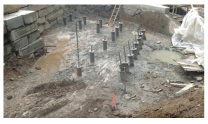
as close as ten feet to the work area, so potential impacts to the brook had to be managed prudently. The work area was contained using tarps, haybales, and other protective measures. Drilling and grouting spoils were 100 percent contained within small local excavations ("spoil pits").
