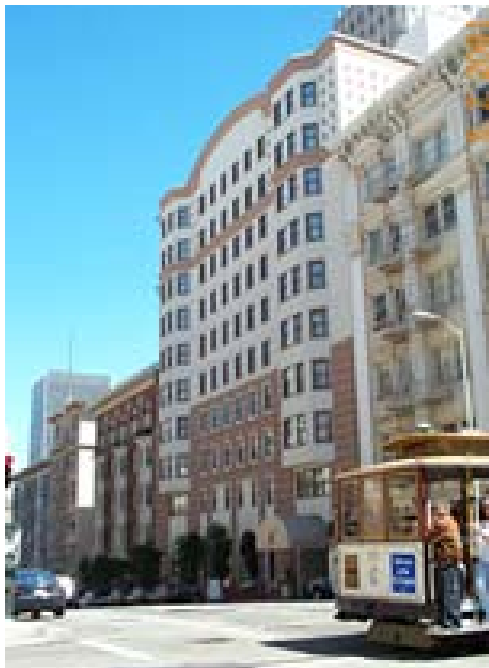
10-story Hotel, San Francisco, CA – Seismic Zone 4
