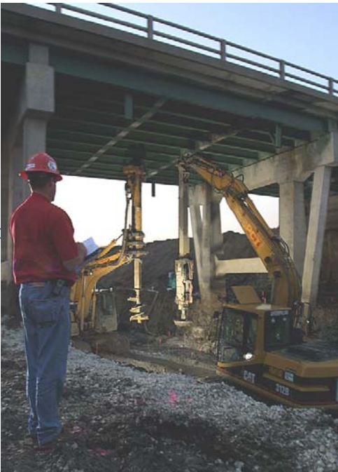
Box Culvert / Embankment Support, Neola, IA
