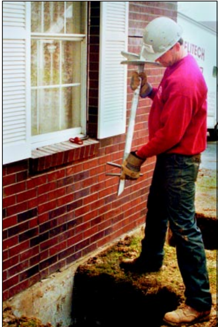
Placing a twin-helix anchor
