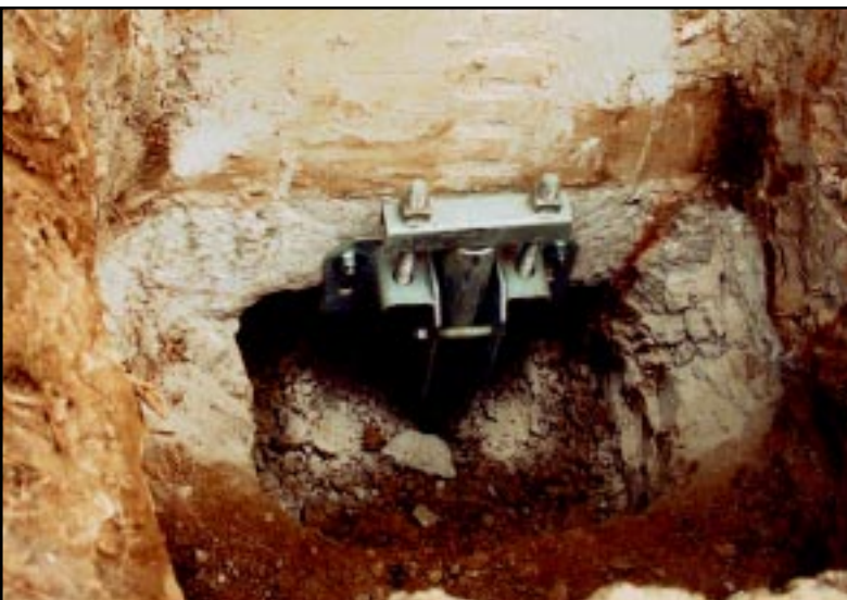
Completed HELICAL PIER® Foundation Systems anchor and bracket
