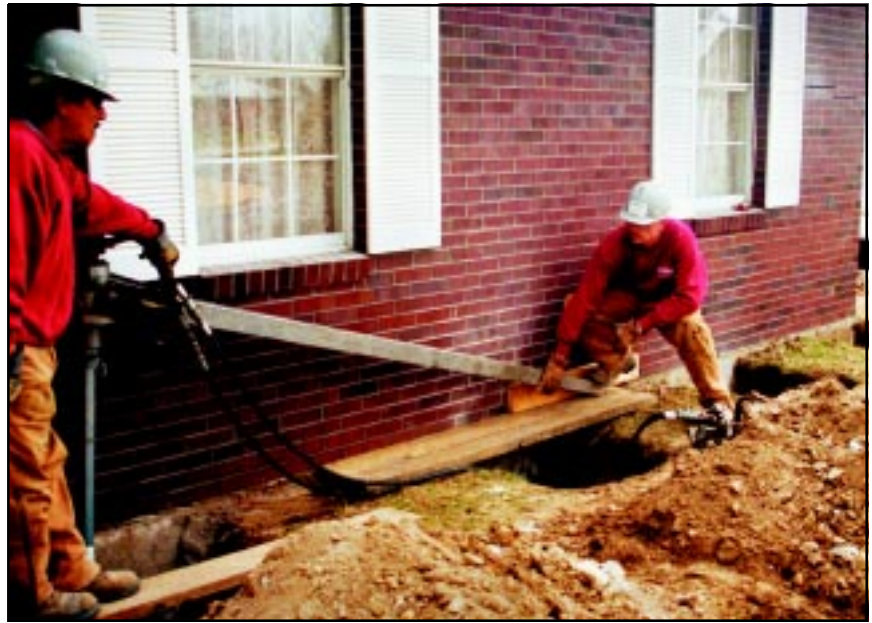
HELICAL PIER® Foundation Systems anchor installation by hand-held hydraulic driver
