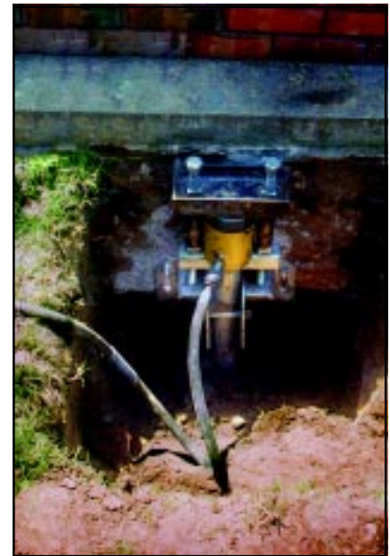
Hydraulic jack pushes down on HELICAL PIER® Foundation Systems anchor shaft and up on foundation held in bracket. After jacking, nuts on top of T-pipe secure the load. Then, jack and plate above are removed to complete installation.
